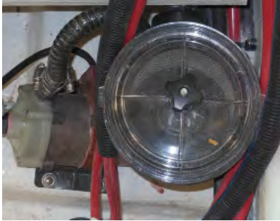
TYPICAL A/C SEAWATER STRAINER/BASKET
